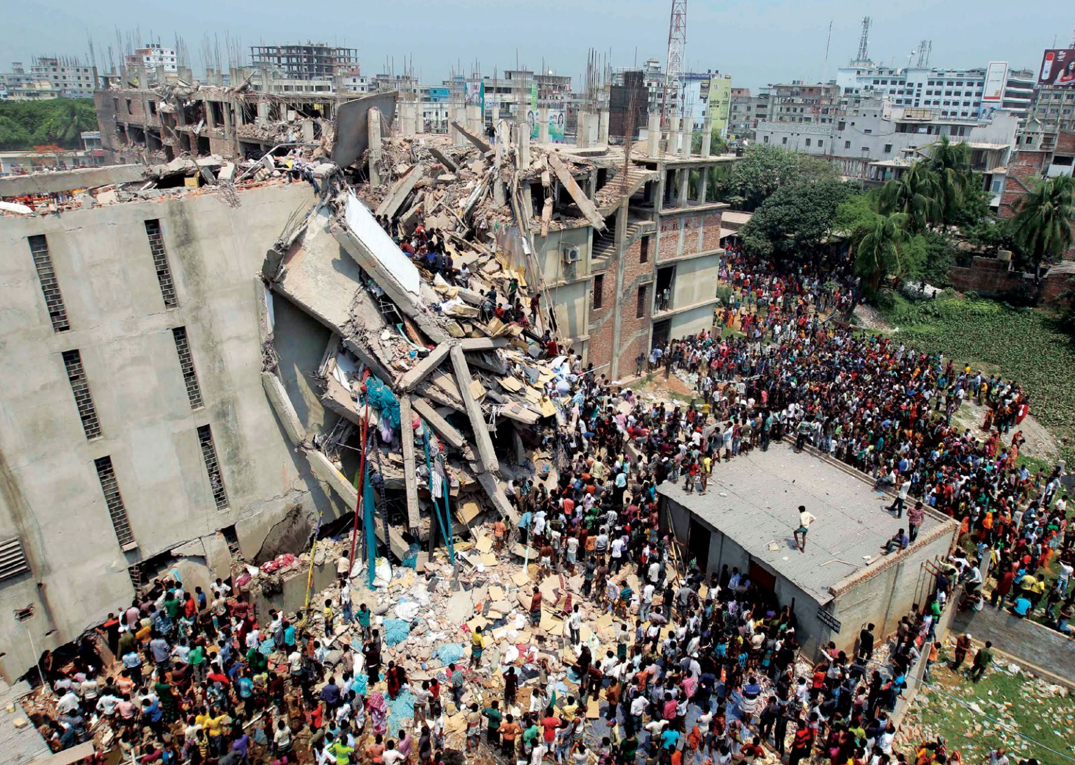
Above: The tragic Rana Plaza factory collapse in Dhaka, Bangladesh, which took more than 1,100 workers' lives on April 24th, 2013.
